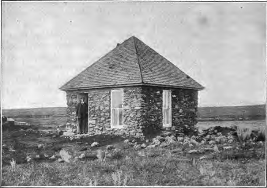
FIG. 157. Stone School-House, Made of (Petrified) Wood, New England, Hettinger County. Photograph by A. L. Fellows.
